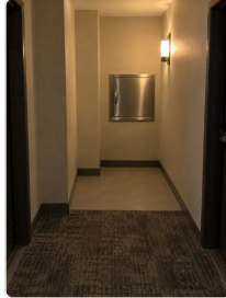
Bldg 12 Floor 3 Trash Chute Clear Sep 27, 7:47 PM CDT
