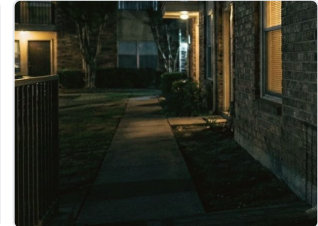
Bldg 10 Breezeway Sep 27, 7:11 PM CDT
